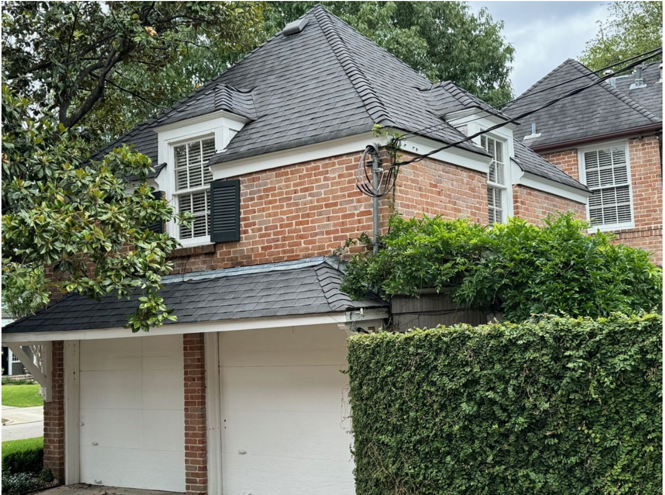
Photo 6: West (side) elevation of the garage and guest living quarters, showing the car garage door access from the side of the lot. Camera facing northeast. Photo by applicant, 2024.
