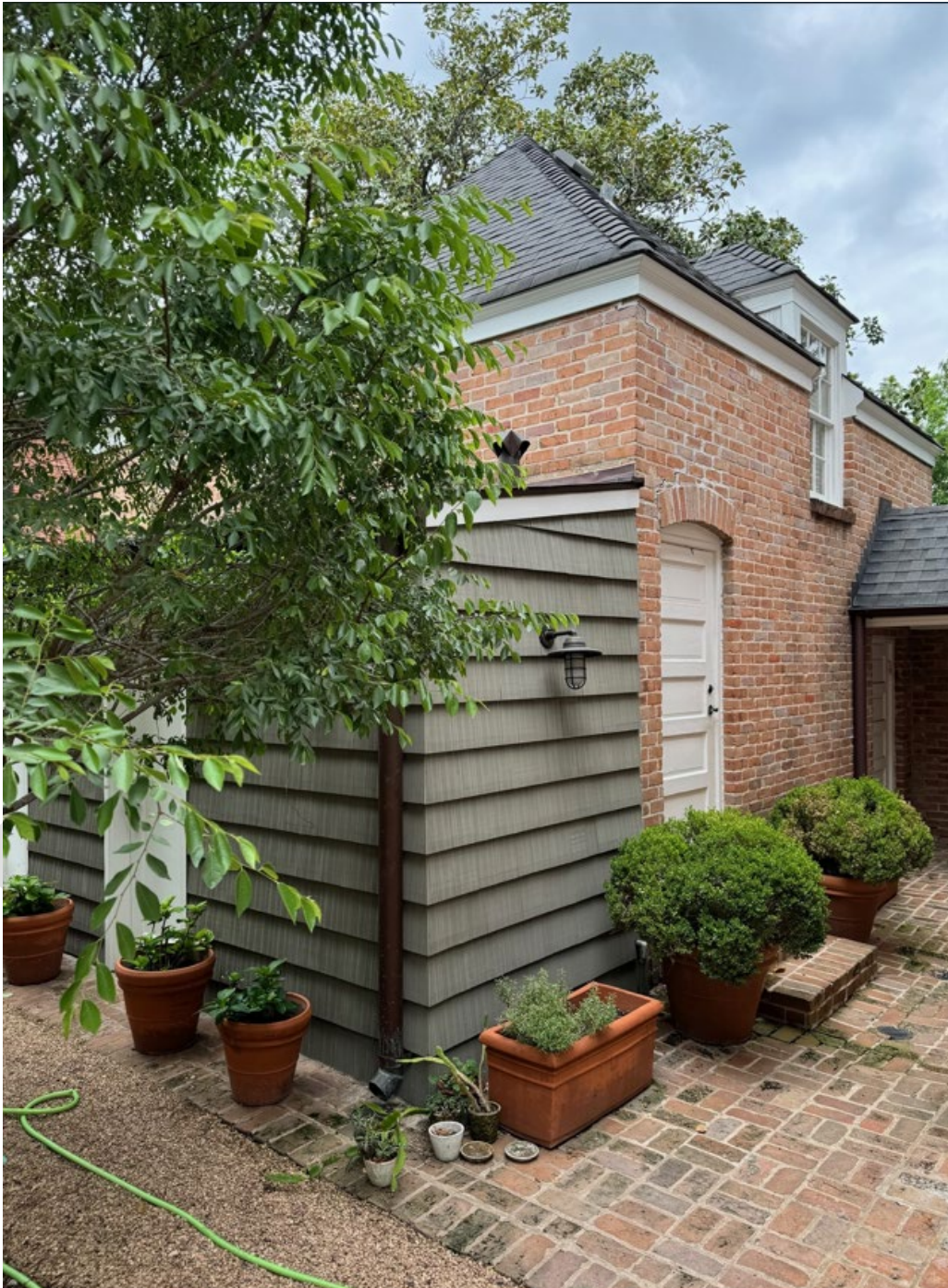
Photo 5: Oblique view of the southeast (rear/side) elevation of detached garage and guest living quarters of the Frank A. Watts House. Camera facing northwest. Photo by applicant, 2024.
