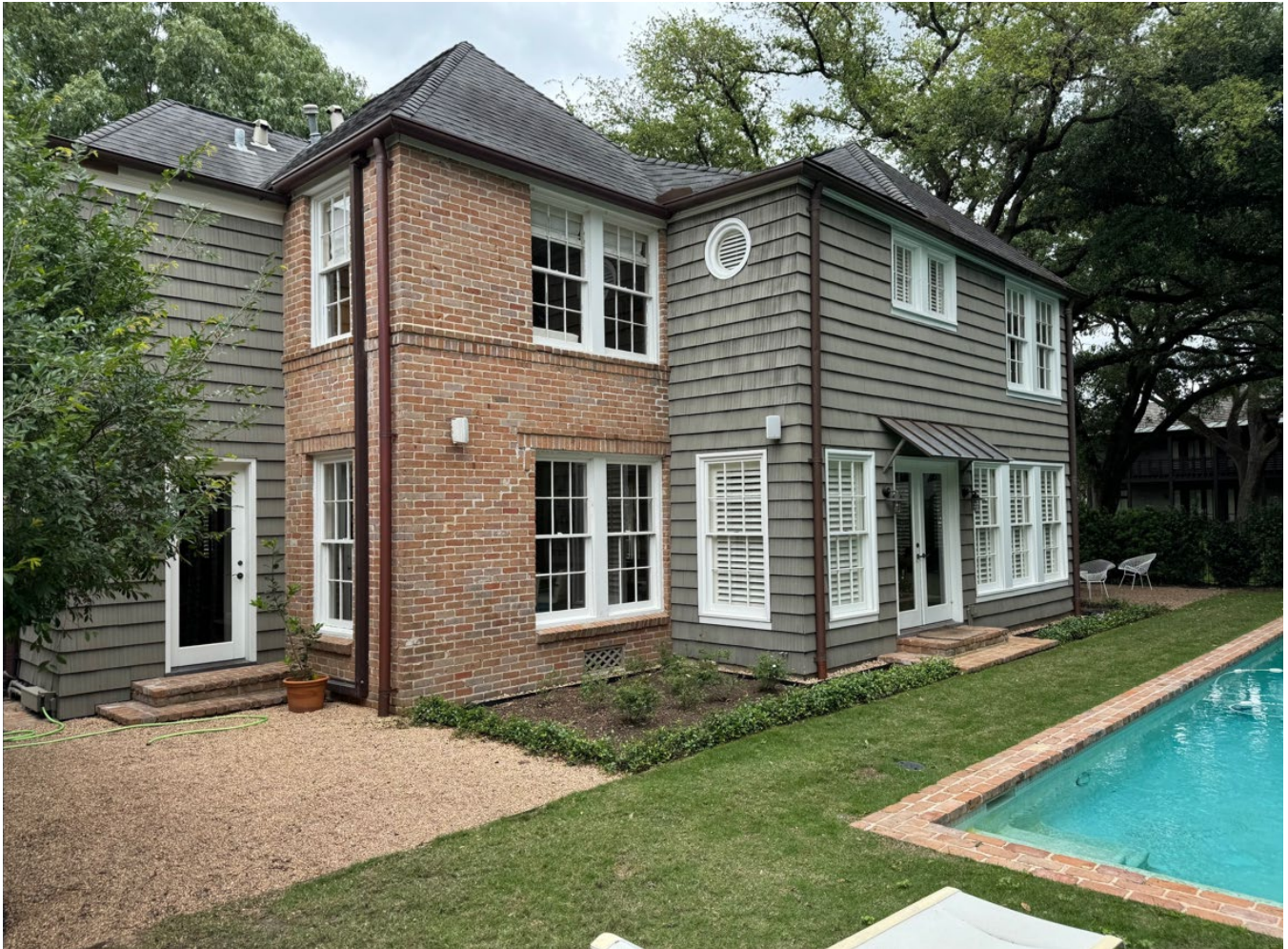
Photo 4: Oblique view of the south (rear) elevation of the Frank A. Watts House, which includes the location of the later wood shingle clad addition. Camera facing northeast. Photo by applicant, 2024.
